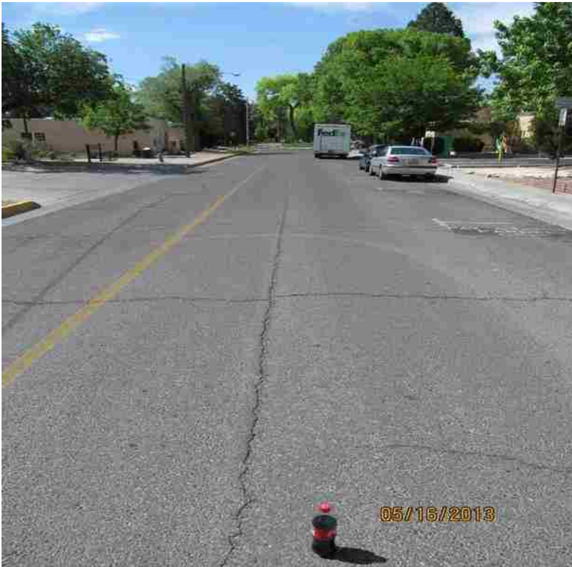
Figure 7. Longitudinal cracking
