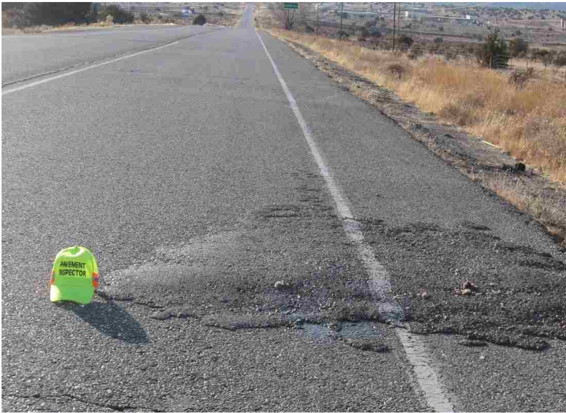
Figure 6. Pavement patching
